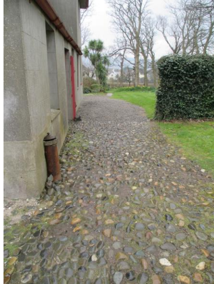
The cobbled path to the rear entrance
