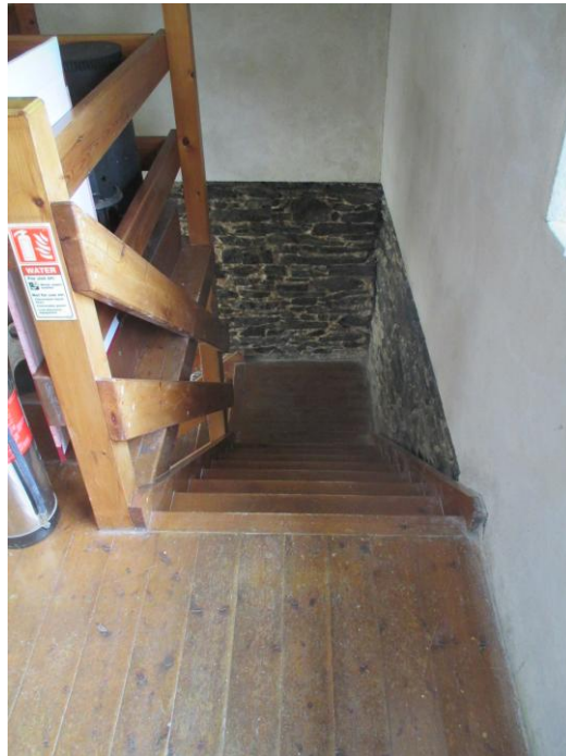
Open-riser steps leading from/to first floor (8 steps with mid-landing)
