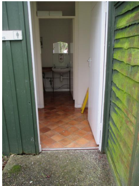
Entrance to ladies toilet (78cm width)
