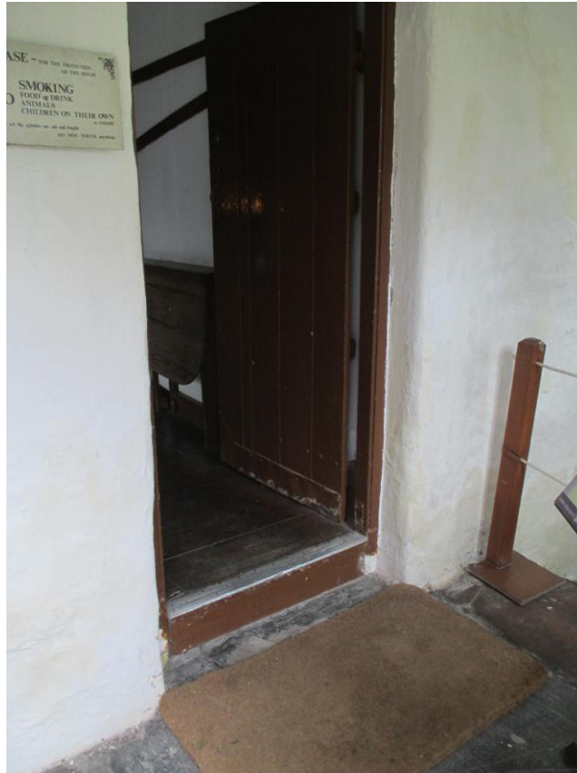
19cm step leading to kitchen back door (doorway 73cm wide)
