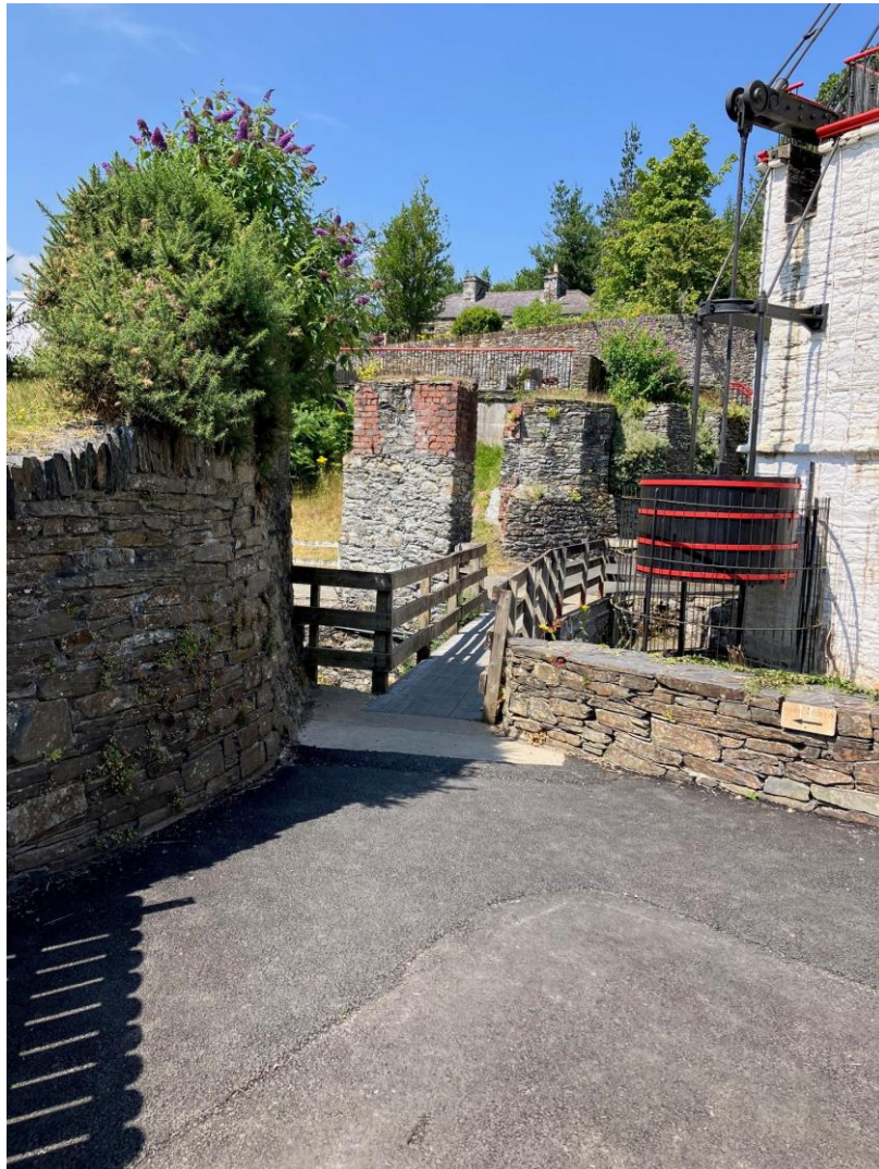
Wooden bridge to base of Laxey Wheel
