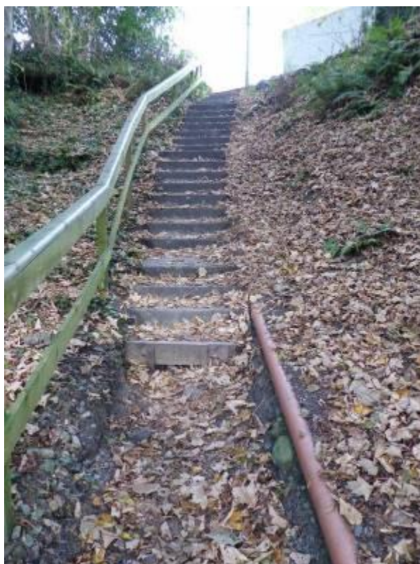
Pedestrian glen entrance from the base of Wheel Hill, showing 28 uneven steps and handrail (3)
