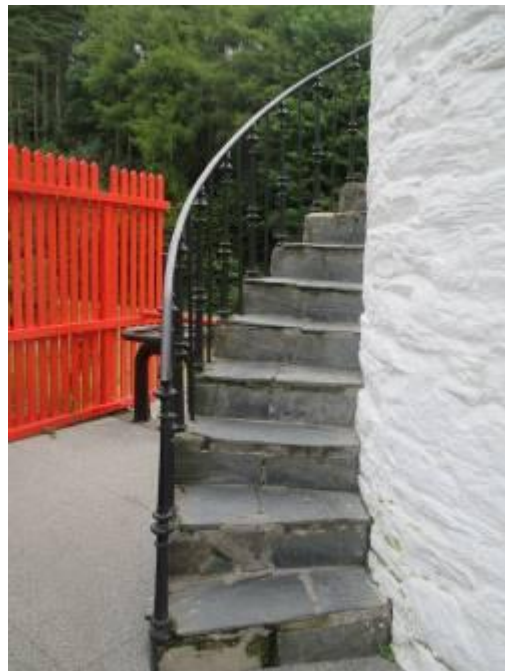
Spiral steps leading to top viewing platform (75 steps)
