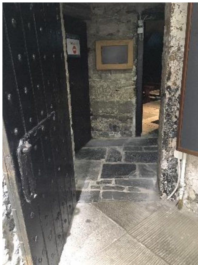
Doorway leading to film room (via small corridor)
