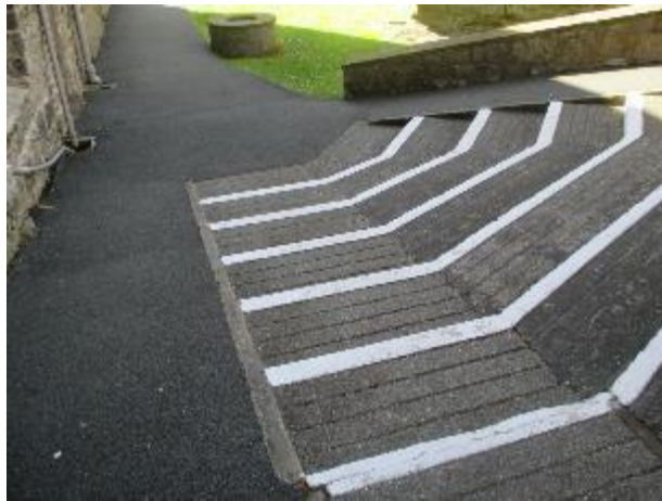
Tarmacked ramped incline leading to the toilet block
