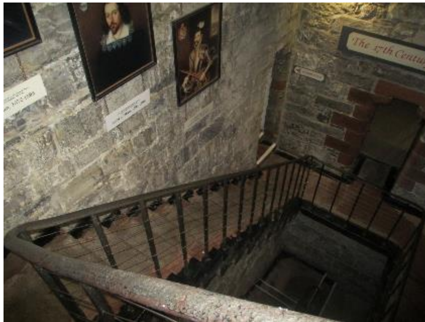
Central stairwell – ‘The Prison Stairwell’
