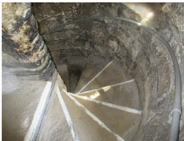
Main spiral staircase
