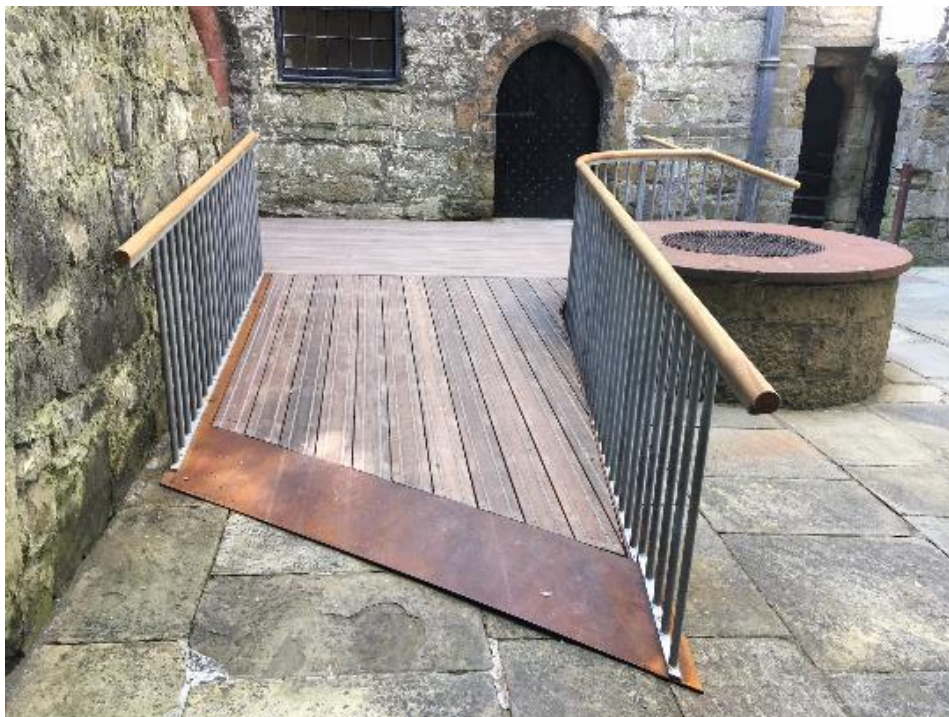
Ramp leading from Courtyard to exhibition and film room – alternatively there are two steps which can be used instead
