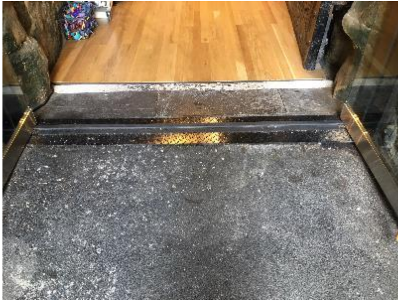
Entrance way showing slight raised lip on door threshold
