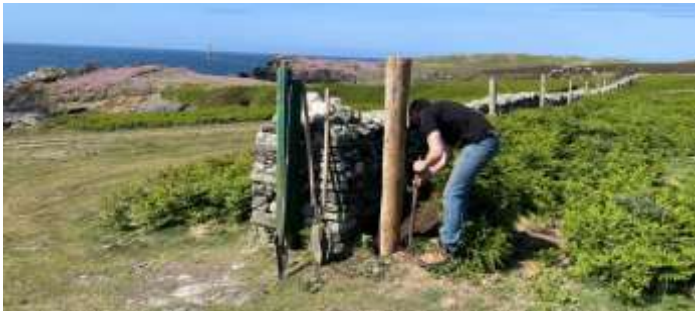
Dom repairing a broken section of fence. ©Kate Fox
