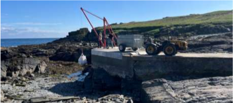
Using the crane to lift a dumpy bag filled with shingle. ©Kate Fox
