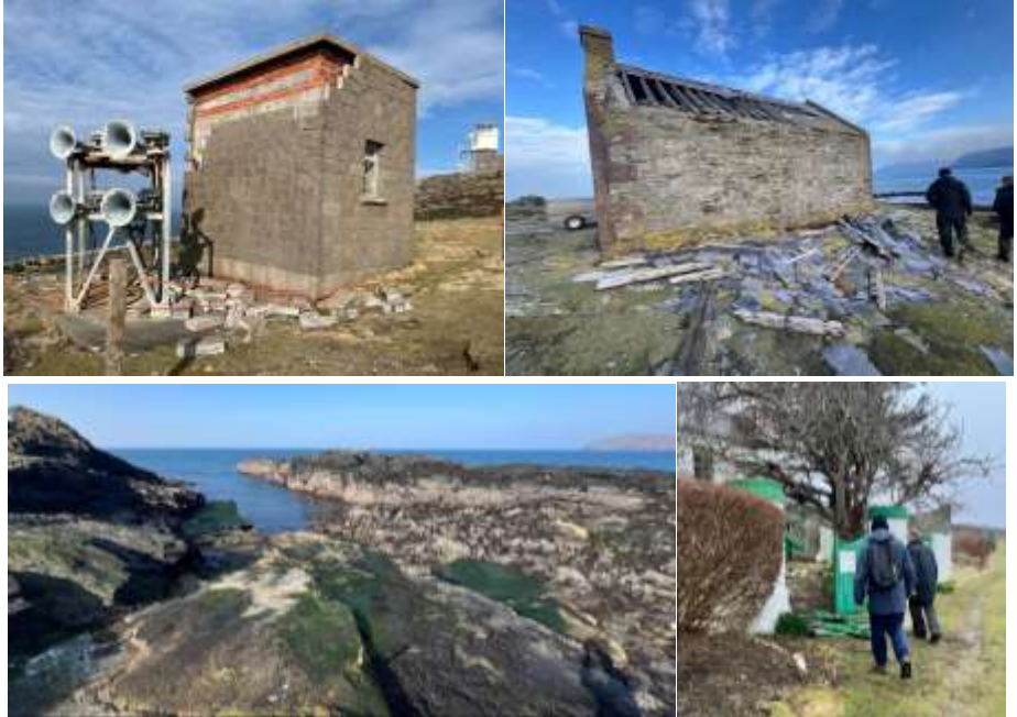
Clockwise from top-left: damage to foghorn building, the Cow store roof, Cow Harbour jetty, and the ruined front gate. ©Kate Fox
