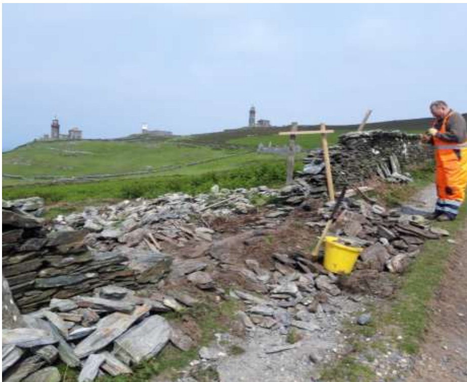
Start of building trackside wall to eastern boundary of lighthouse fields (June 2024)
