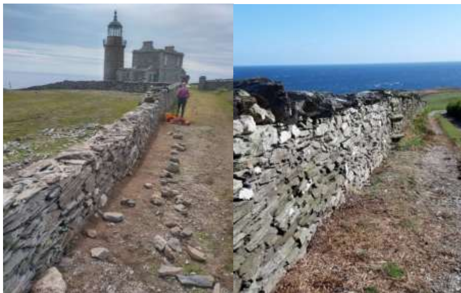
Wall on approach to Lower Lighthouse – part completed (June 2022) and completed trackside wall to eastern boundary of lighthouse fields (June 2024)
