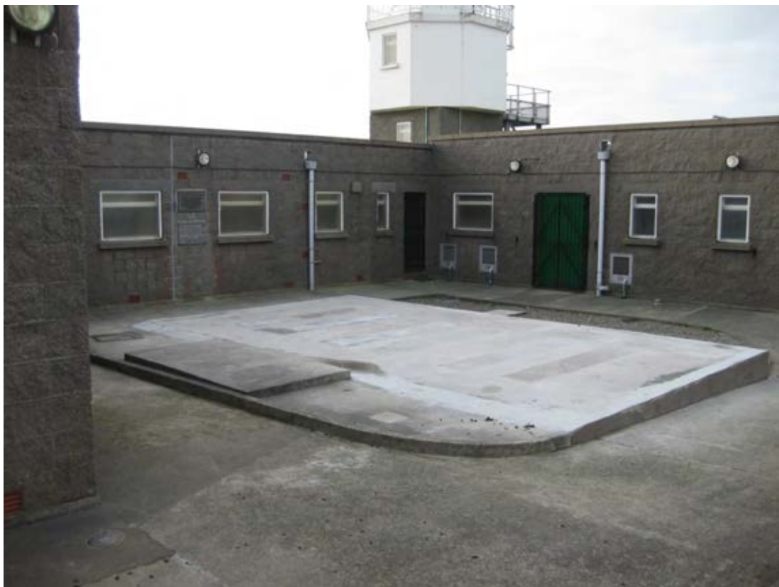
1968 Lighthouse – Before and after removal of diesel tanks (Photos: Shaun Murphy)
