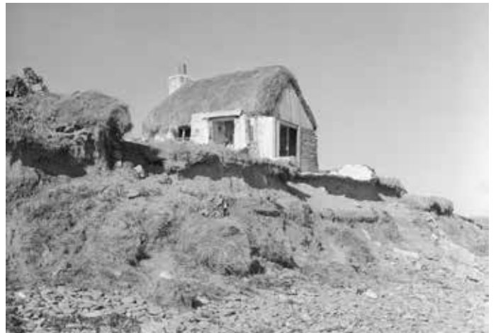
Thatched cottage and coastal erosion, Bride, 1965.
