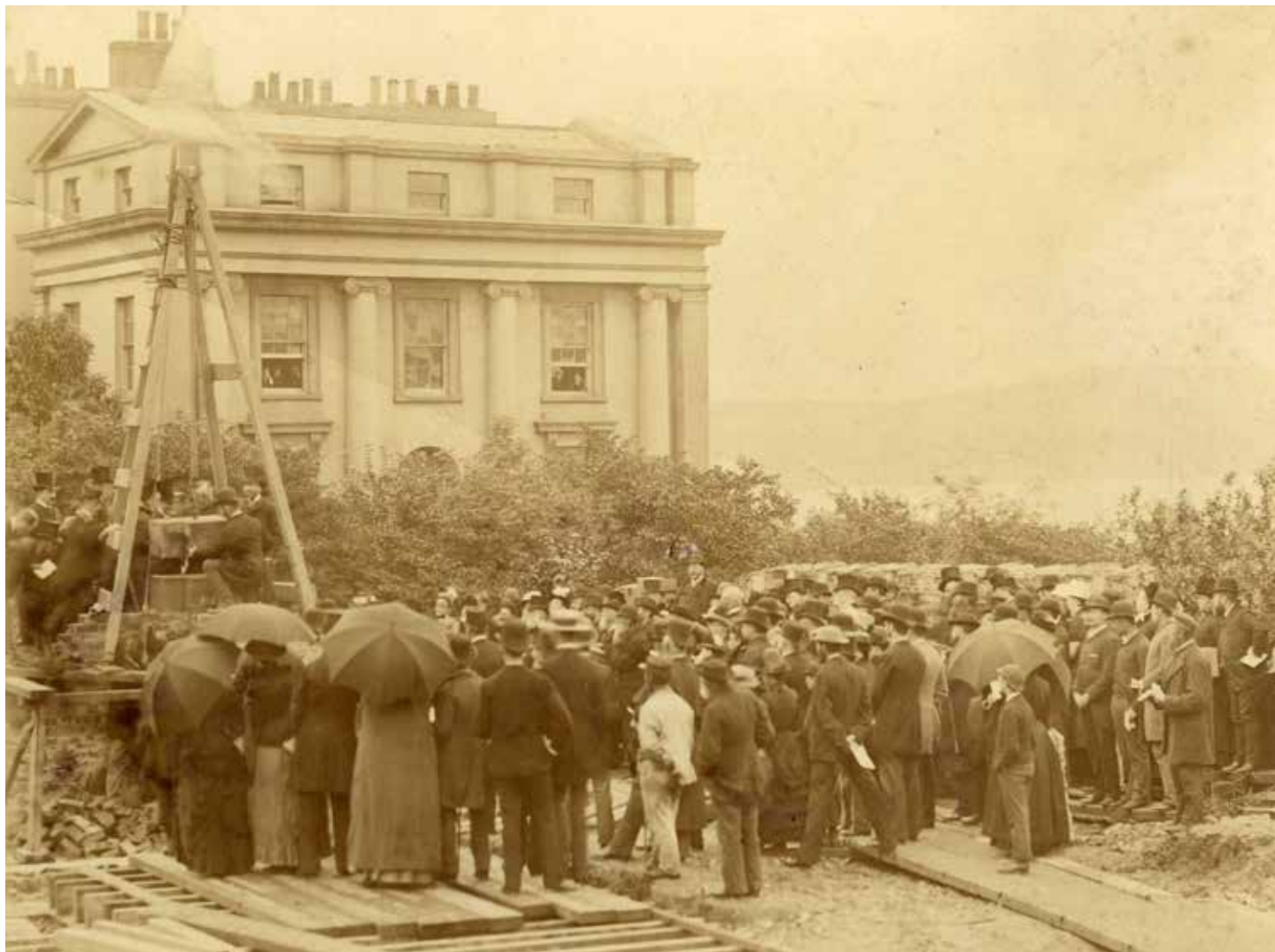
Laying foundation stone of Noble's Isle of Man Hospital, Douglas on 26 July 1886.
