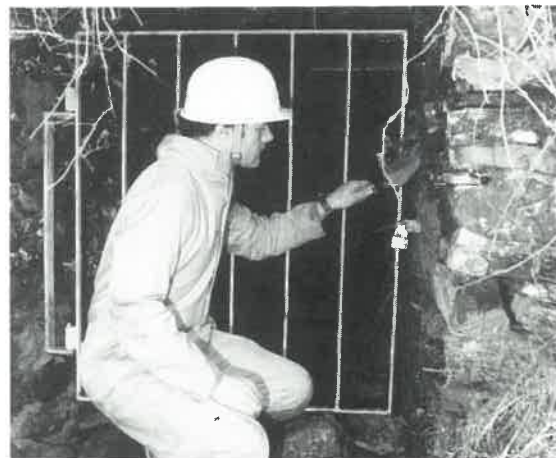
A dangerous mine entrance is sealed. Glen Rushen.
