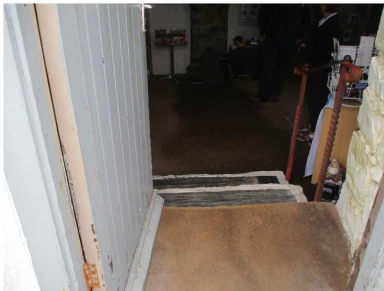
Showing entrance and steps
