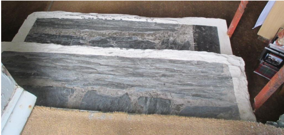
Close up detailing the steps
