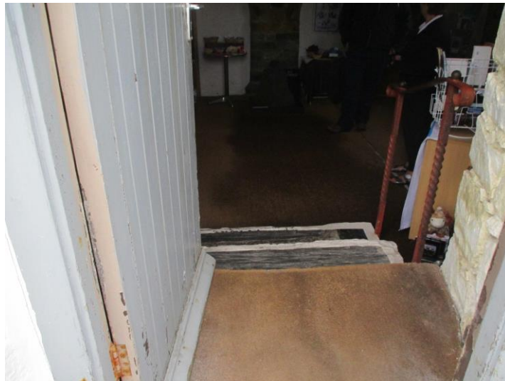
Showing entrance and steps
