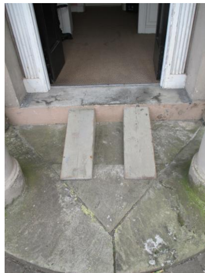
Main entrance – detailing temporary ramp
