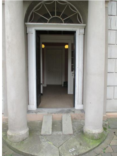
Main entrance – showing moveable wooden ramps and slight step
