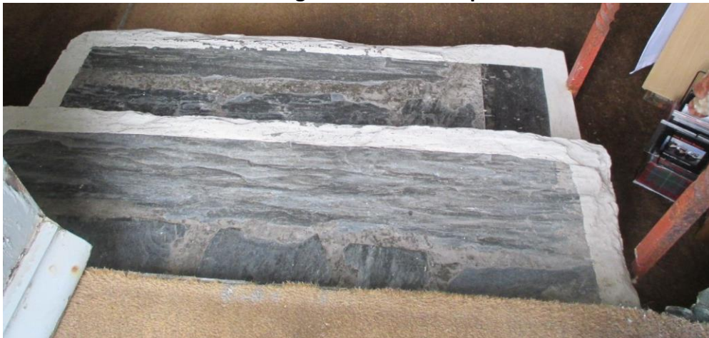
Close up detailing the steps
