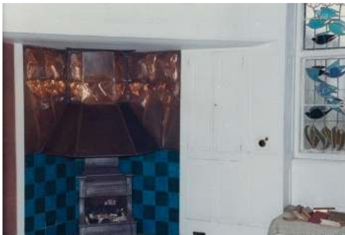
Hall at Glencrutchery House.
