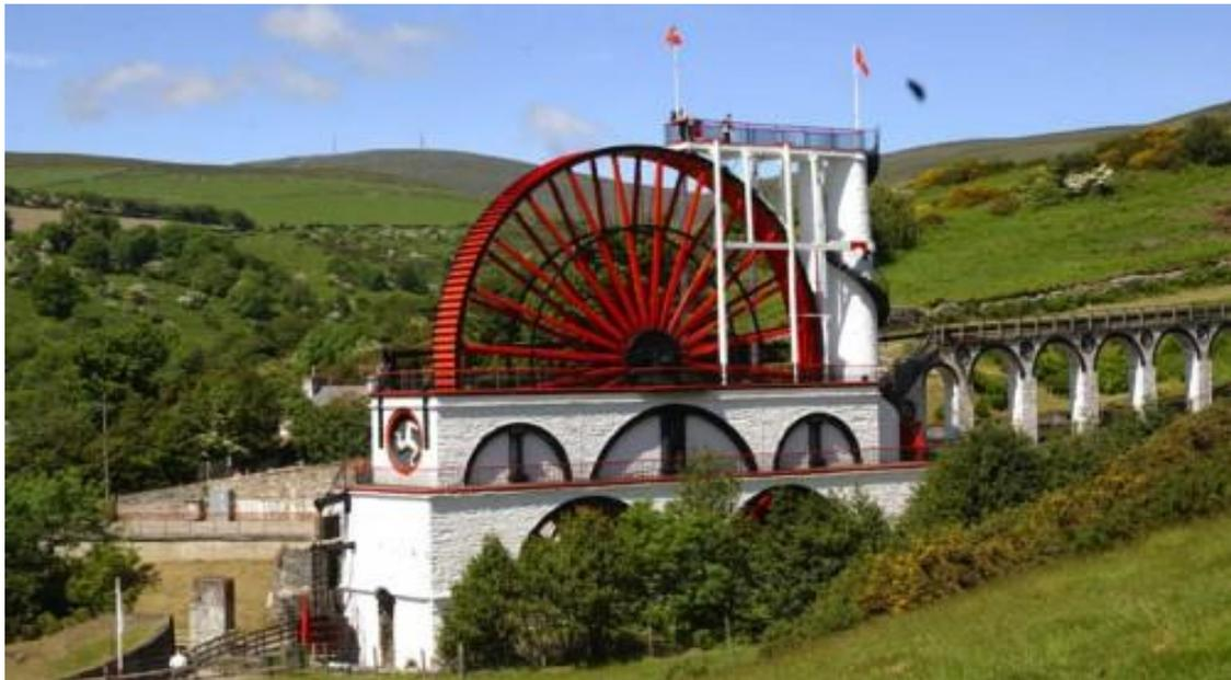
The Great Laxey Wheel is the largest surviving working waterwheel of its kind in the world. Designed by the Victorian engineer, Robert Casement, the wheel was built in 1854 to pump water from the Glen Mooar part of the Great Laxey Mines industrial complex.
